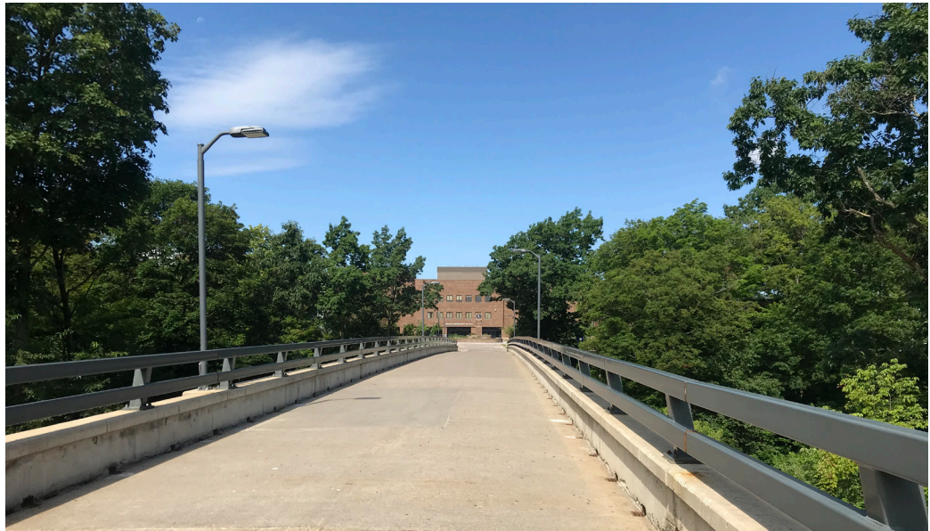
Campus Pedestrian Bridge
